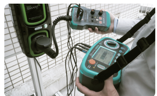
Photo of EVSE charge point testing by EVSE ADAPTER and MFT
